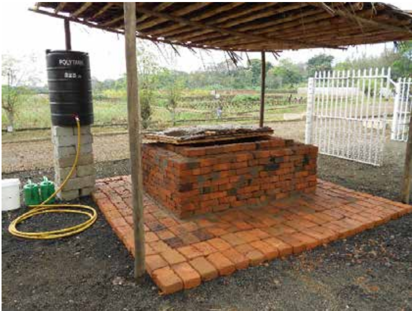
Improved zero-energy cool chamber (ZECC) with water supply and shade cover in Arusha, Tanzania. Photo courtesy of Lisa Kitinoja/Postharvest Education Foundation
